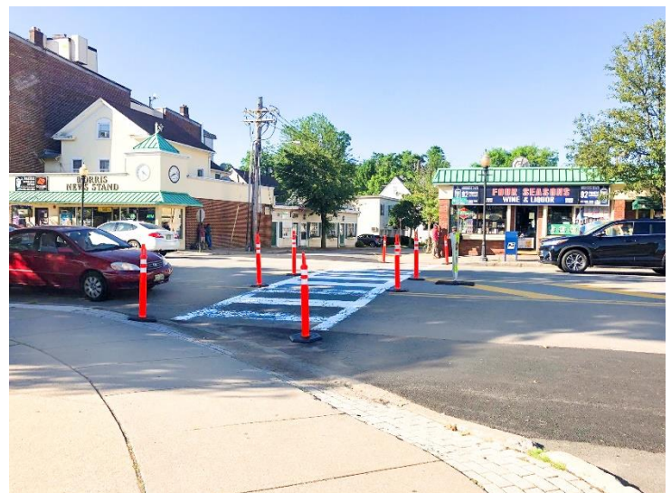
Temporary Delineator Set-Up at Morris Street and King Street
